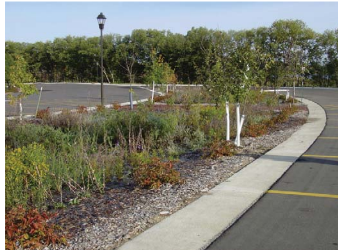
Bioswale collecting parking lot stormwater
