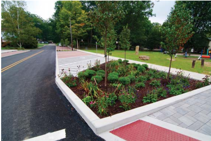
Bioswale bumpouts and pervious paver parking stalls (Ohiopyle, PA)
