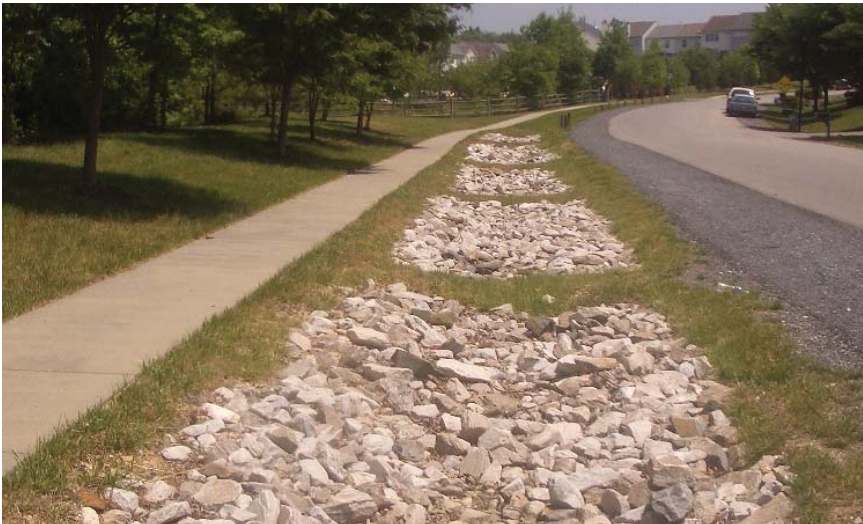
These small basins are linked to collect water from the adjoining road
