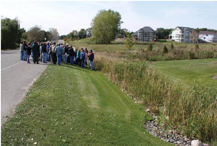
Bioswale collecting roadway stormwater
