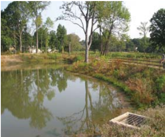
Small wet pond in a park with overflow structure
