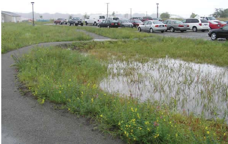
Bioretention pond collecting stormwater from the parking lot
