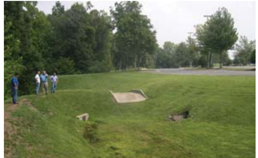
Large dry detention basin with decorative plantings
