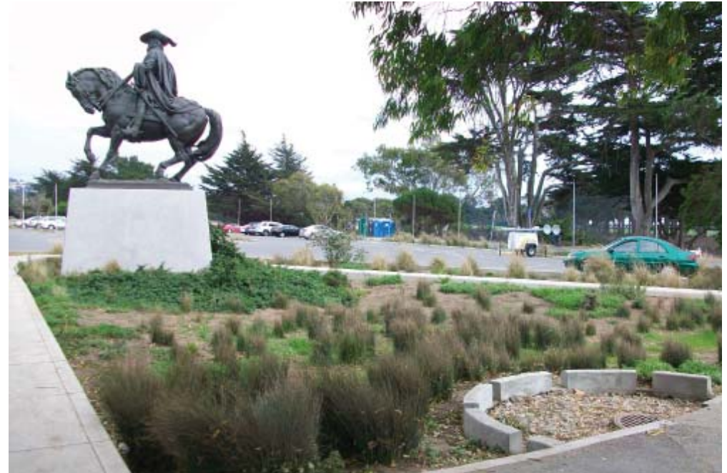
Urban infiltration basin with sediment trap
