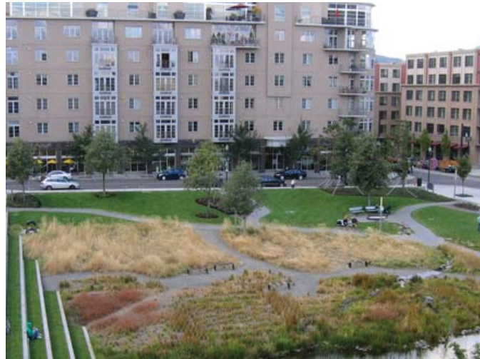
Stormwater wetland in an urban setting
