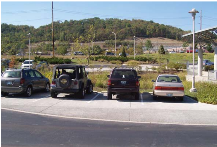
Pervious concrete parking stalls (Louisville, KY)
