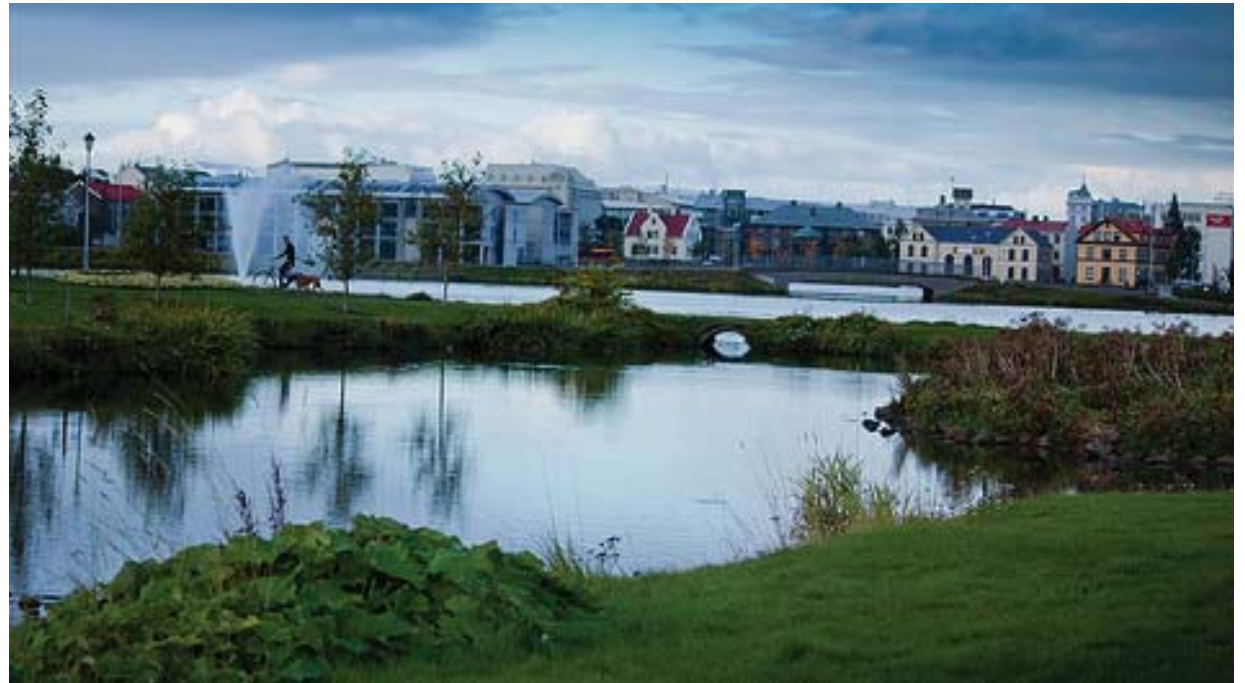
A series of wet ponds can be linked together to provide for maximum storage such as this urban wet pond
