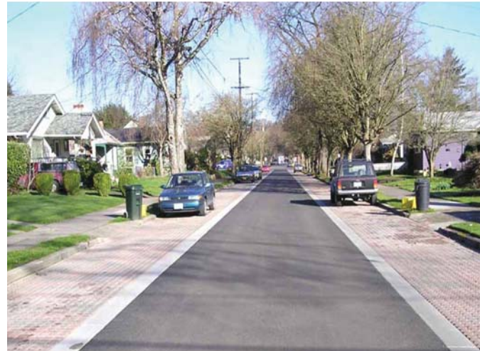
Pervious paver on street parking stalls
