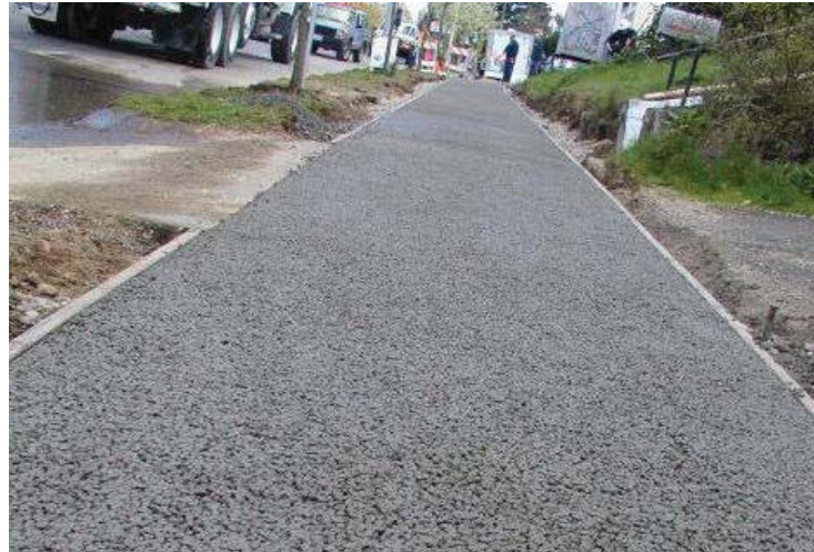
Permeable concrete used as a sidewalk
