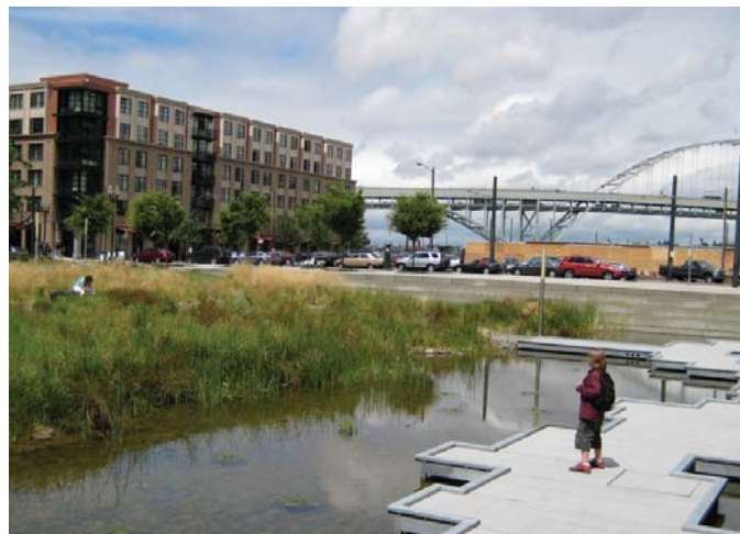
Stormwater wetland in an urban setting
