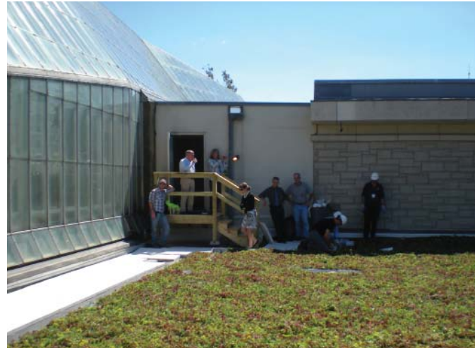
Tray green roof installed by volunteers (Cleveland, OH)
