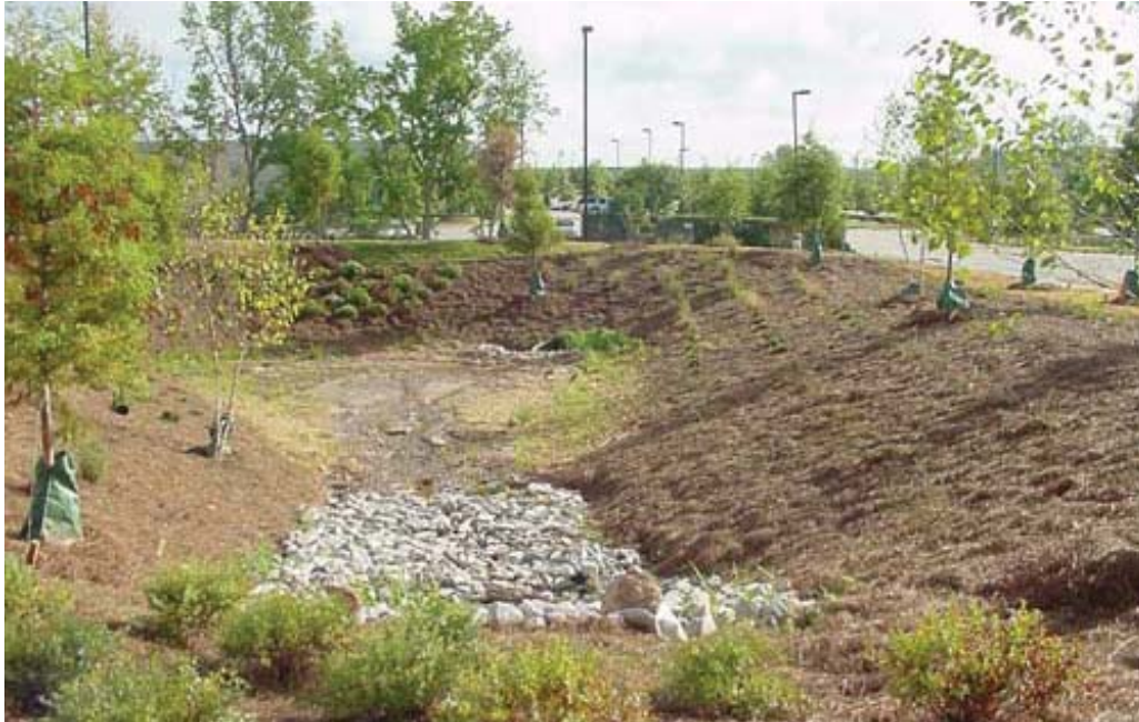
Small dry detention basin
