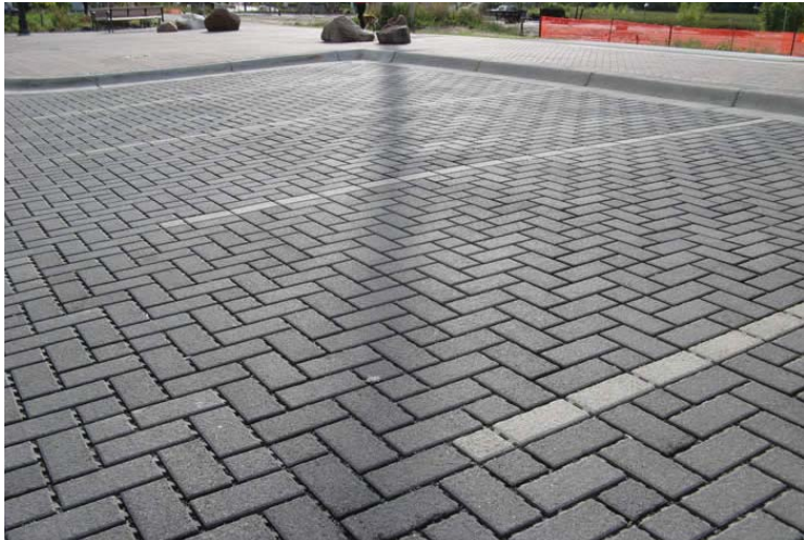
Permeable concrete pavers used in parking stalls
