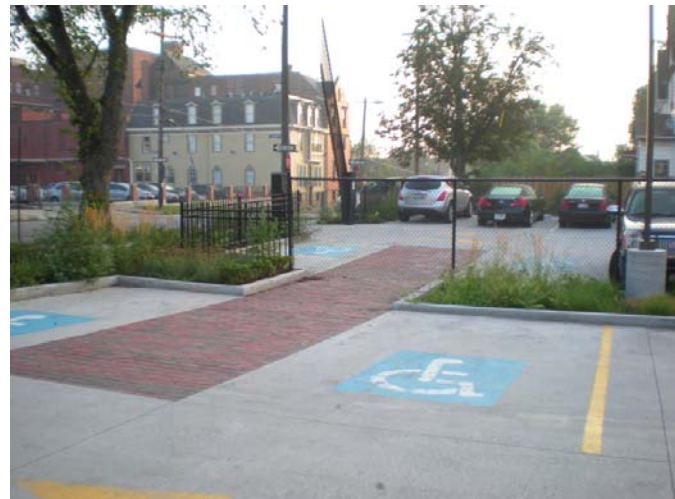
Bioswale with pervious paver handicap aisle (Cleveland, OH)
