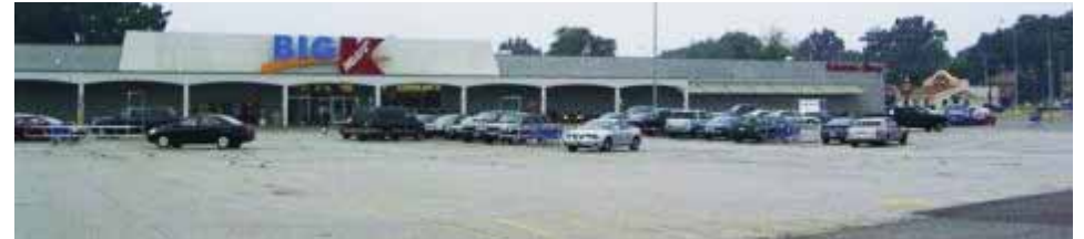
Example of large directly connected impervious area
