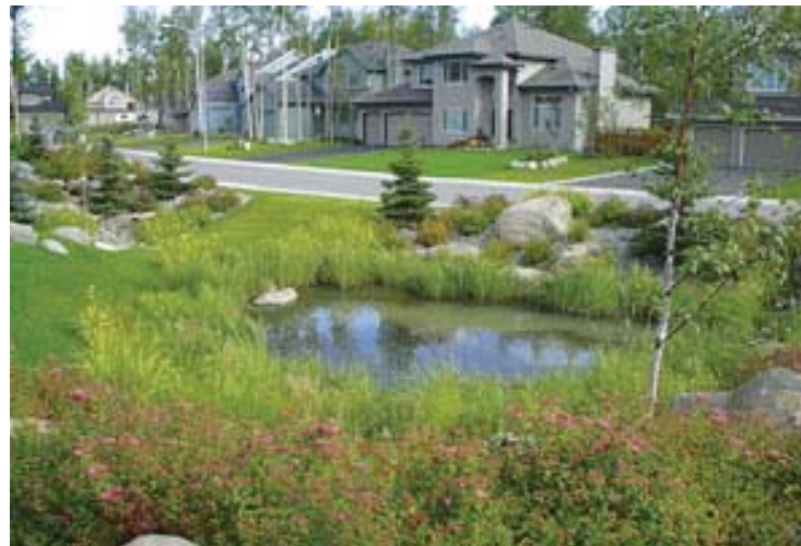
Bioretention pond collecting stormwater from the street
