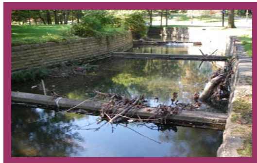
Concrete Check Dams ▼
