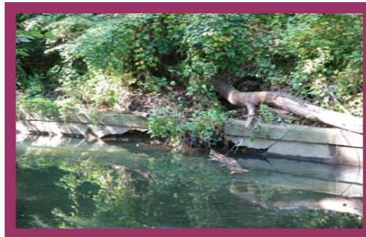
Failed Concrete Wall ▼
