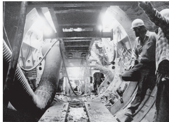
Drilling begins on the Southwest Interceptor (Contract 5), 1989
