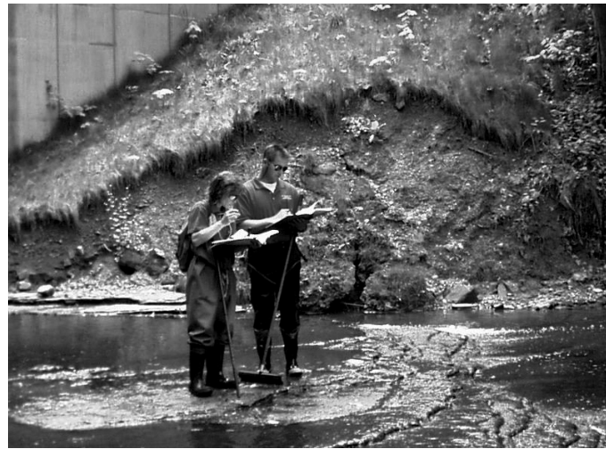
The Regional Plan for Sewerage and Drainage included inspections of local streams to document problem areas, such as this 2004 example of bank erosion along Euclid Creek.
