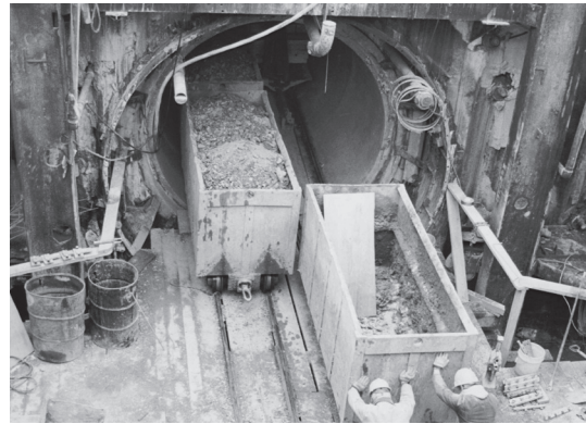
Mining cars remove debris during construction of the Heights/Hilltop Interceptor, 1988
