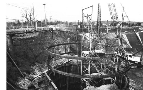
Cuyahoga Valley Interceptor Lift Station, 1978
